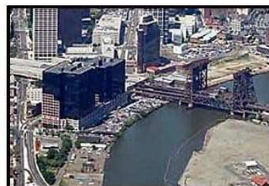
1995 Penn Plaza and Railroad Bridge
